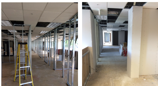
DTC OFFICE IN PROGRESS
